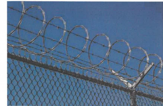
NOT PERMITTED: Wire mesh & razor wire
