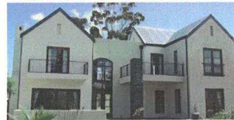
PERMITTED: White painted walls
