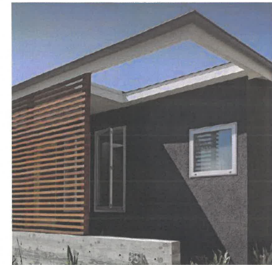
NOT PERMITTED: Dark paint over more than 15% of façade
