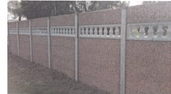
NOT PERMITTED: Vibracrete fence
